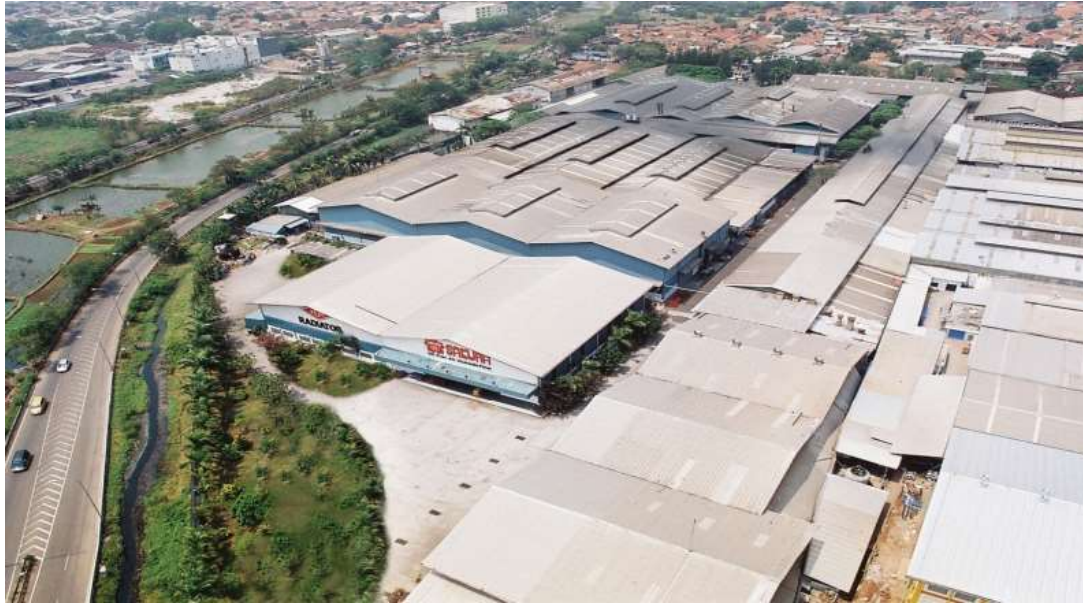
Kapuk Plant (Radiator Facilities)
